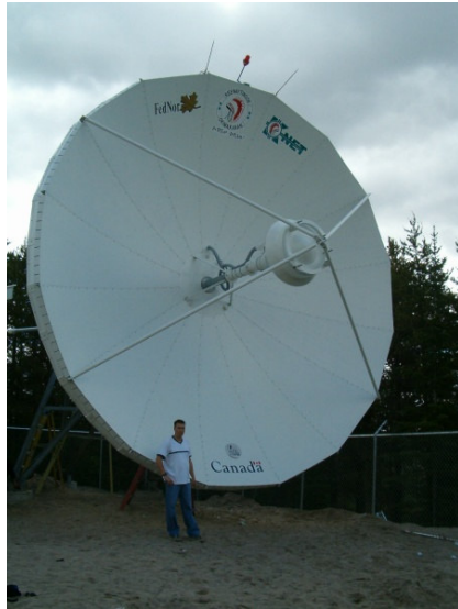
Figure 7. The “Big Dish”, a 7.3 metre satellite earth station located at Sioux Lookout. The earth station is part of K-Net's facilitation of the C-Band Public Benefits Transponder, a joint project with Telesat and Industry Canada.
